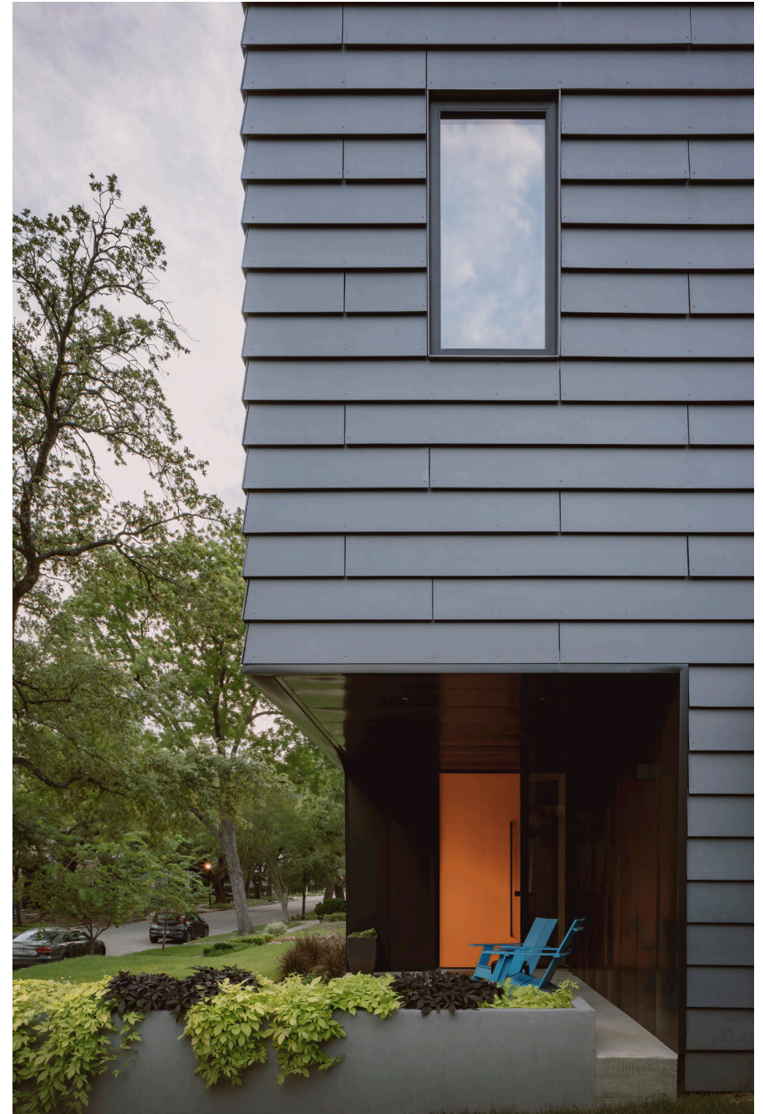
a furring strip exaggerates the depth of the fiber cement lap siding, paying homage to the cladding of the traditional bungalows
