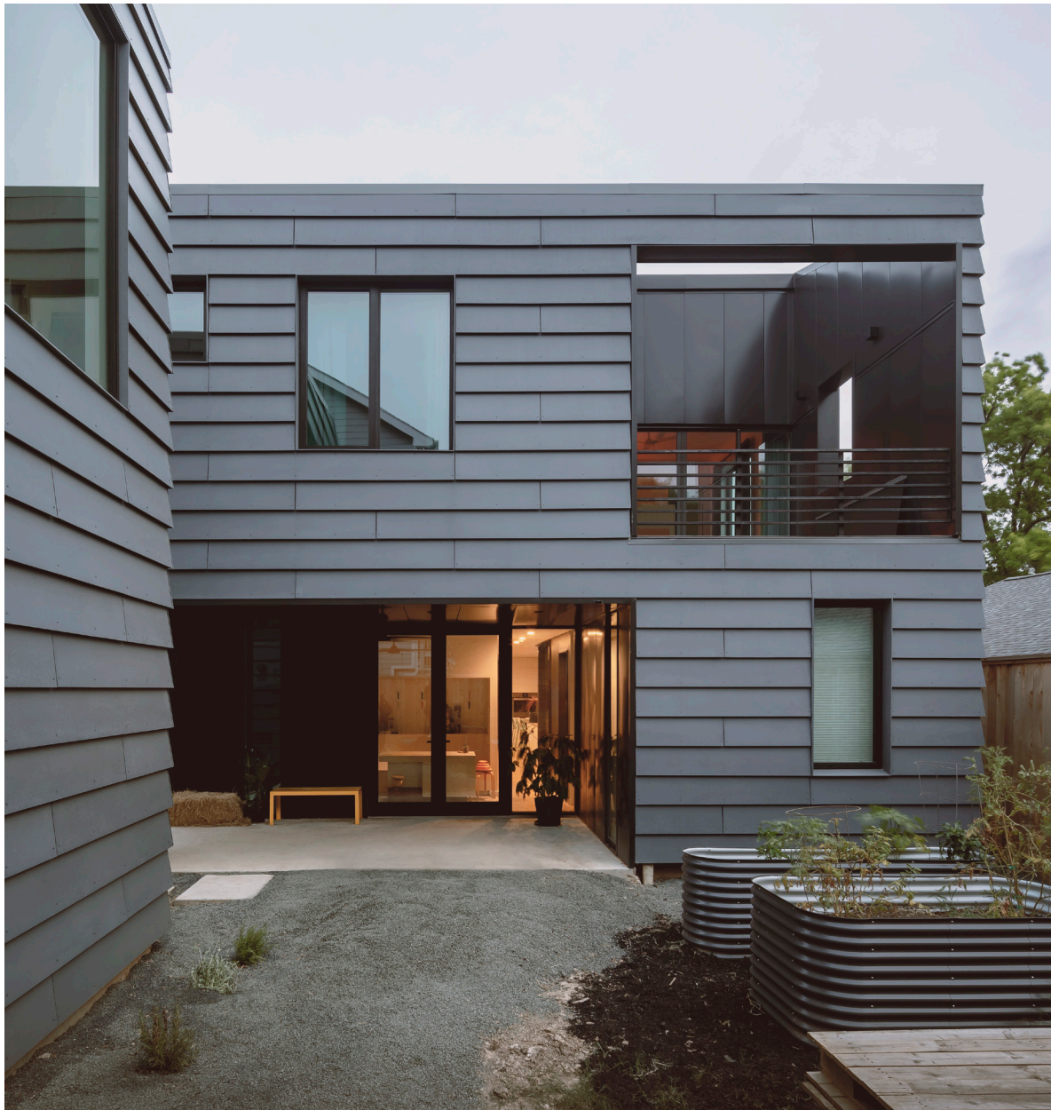
dark metal panels define the exterior patios at the front porch, back porch, and off each bedroom
