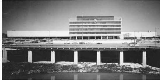
The downtown Post Office under construction (1959)
