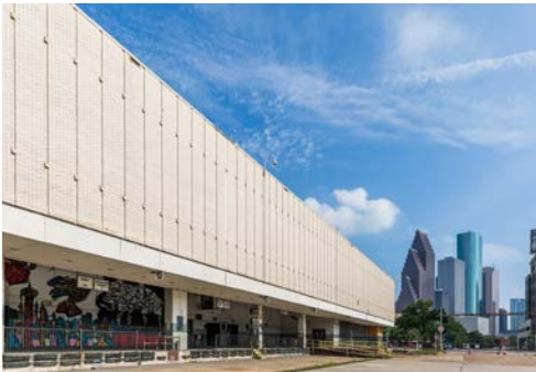
North facade, before
