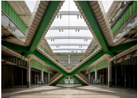
A zigzagging stair is reflected to create adouble “X” with two floating intersections.
