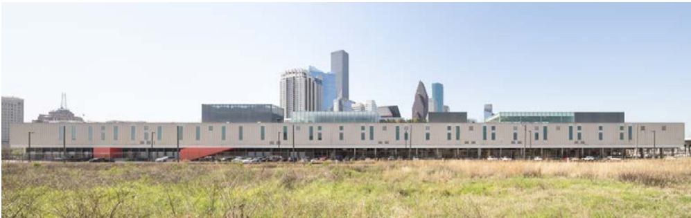
The fundamental character of the original facade is preserved by transforming existing vents into windows and interspersing existing openings with floor-to-ceiling windows of the same width.
