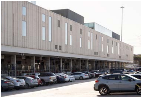
North facade, After
