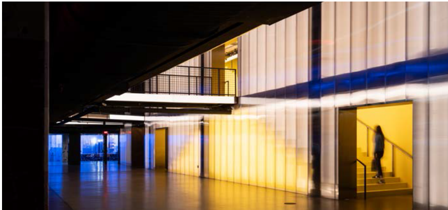
Beyond the lobby, a double-height polycarbonate wall forms a translucent threshold dividing the main space into two zones—a circulation band and the general assembly.
