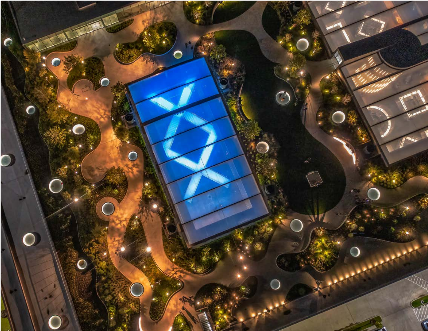
Each atrium is capped by a lightweight air-filled plastic pillow that lets abundant natural light into the offices, shops, and food stalls. A network of skylights across the Skylawn' bring light into the tenant zones and interstitial spaces.
