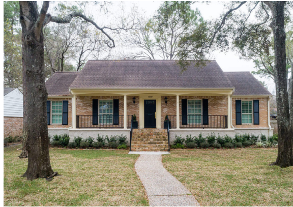
typical response to flooding traditional home elevated above the flood plain and placed on a plinth with crawl space below
