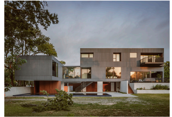
our response to flooding contemporary home elevated to provide shaded outdoor living space and connections to landscape
