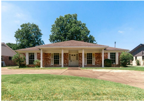
traditional home slab on grade construction with minimal elevation that leaves home prone to increased flooding
